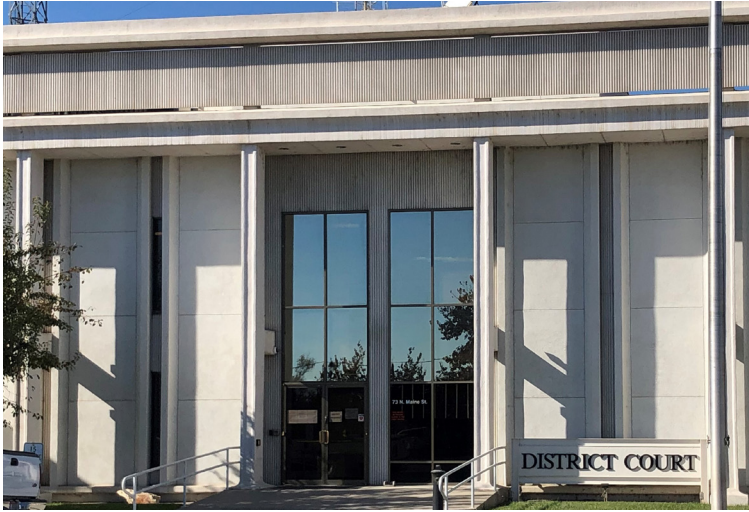
Front of District Court building. Photo by Anne McMillin
