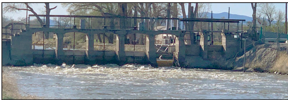
V-Line Canal water levels continue to rise. Photo by Leanna Lehman.
